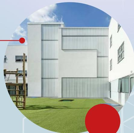
At **Queensmill School**, Linit Glass was used as both main cladding elements and in combination with a metal panel system to maximise natural light into the classrooms.
