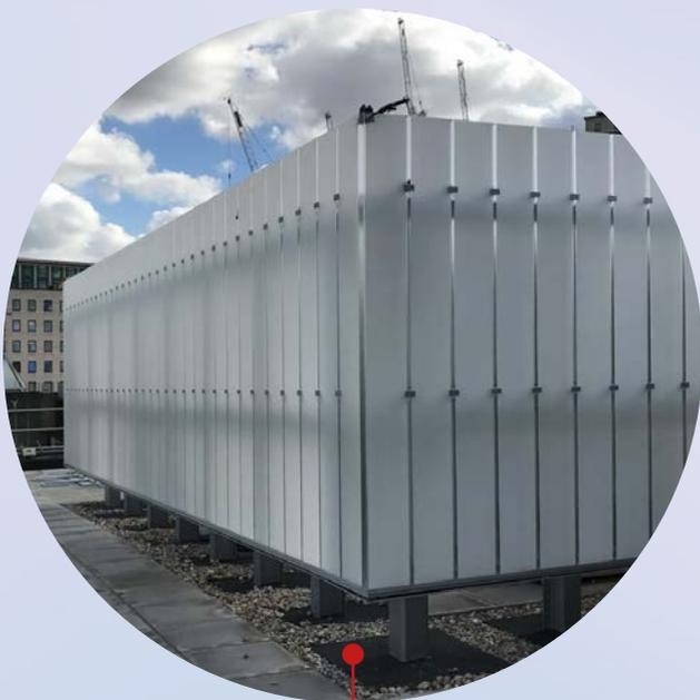
The ability of the Linit Glass system to be installed open jointed has resulted in its use across numerous buildings as a rooftop plant screen. At the **Southbank Centre**, the rooftop equipment is concealed behind a glass screen which allows ventilation to the equipment for air intake and cooling, while providing an aesthetic crown to the top of the building.
