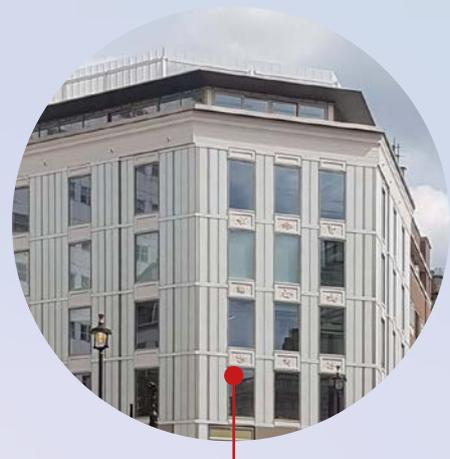
**Sussex House** was the renovation and recladding of an existing building near Leicester Square which combined Linit feature panels with stone cladding and strip windows. The combination of the Linit panels and the strip windows enhanced the natural light being allowed through to the interior floors while also providing an amount of privacy.
