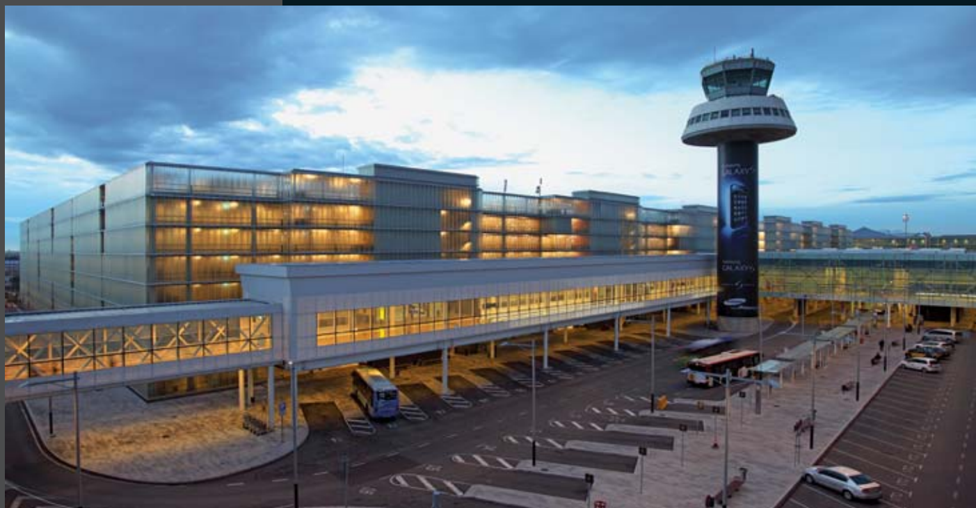
AIRPORT BARCELONA PARKING BARCELONA, E
