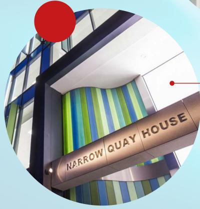
At Narrow Quay House in Bristol, a different bar code effect was created using different enamel colours on the glass in addition to the sweeping S-Curve giving a very distinctive look to the main entrance of the building. The enamel paint is available in any RAL colour with an endless number of combinations that can be achieved.
