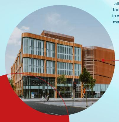
At Broadmarsh Car Park, the Linit Glass system was used to create an open jointed façade with sweeping bullnose corners and curves. The three different glass surface finishes combined with an enamel paint finish enabled the design team to create a randomised bar code across the façade while providing the ventilation required to the car park interior and avoiding the need for air extraction systems.
